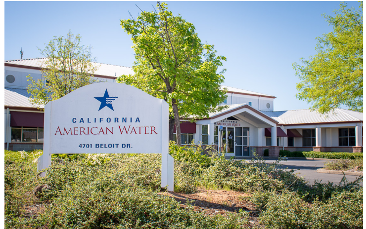
California American Water installed AMS's online, MetalGuard Cr(VI) analyzers, which allowed it to monitor and address critical steps in its remediation process.
