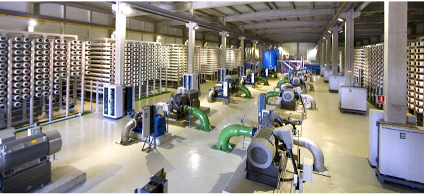
RO Membrane System at Sant Joan Despí DWTP
