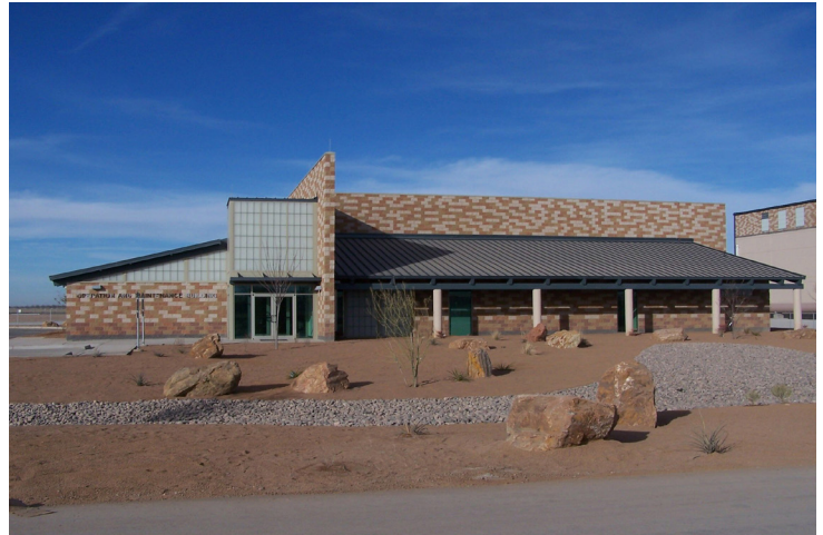
El Paso Water's Upper Valley Water Treatment Plant installed three automated online arsenic analyzers, which provide high-frequency, real-time data on arsenic contaminant levels in 30 minutes with sensitivity down to 1 ppb.
