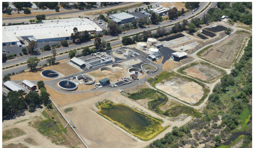
City of Paso Robles Wastewater Treatment Plant
